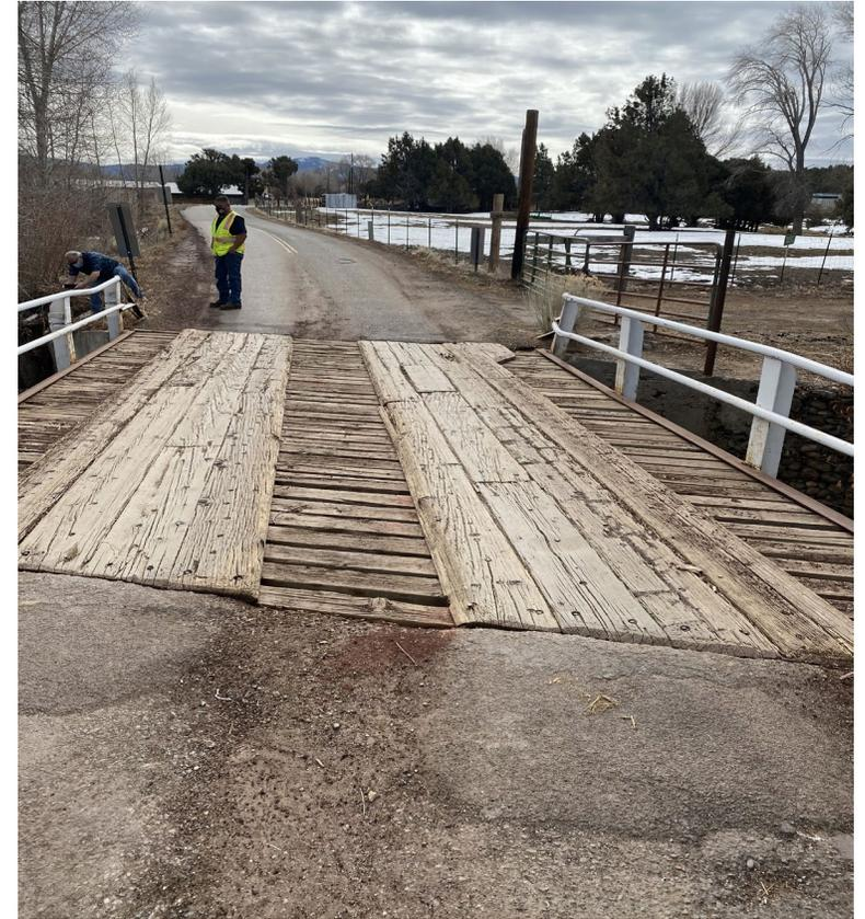
Visual signs of deterioration of timber plank decking due to ultraviolet light and high moisture conditions
