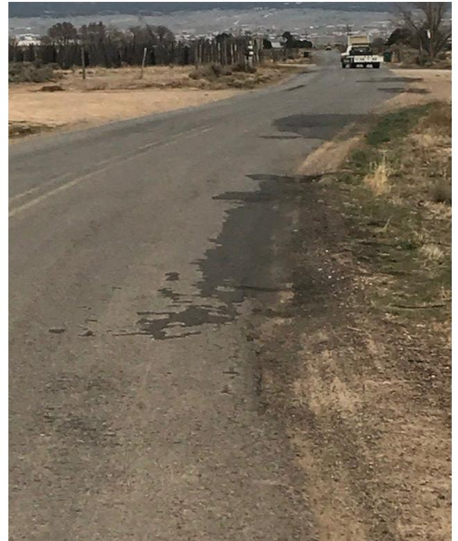
**Open raveled alligator cracking with settlement along lane edge most likely due inadequate subgrade and commercial traffic loads.**
