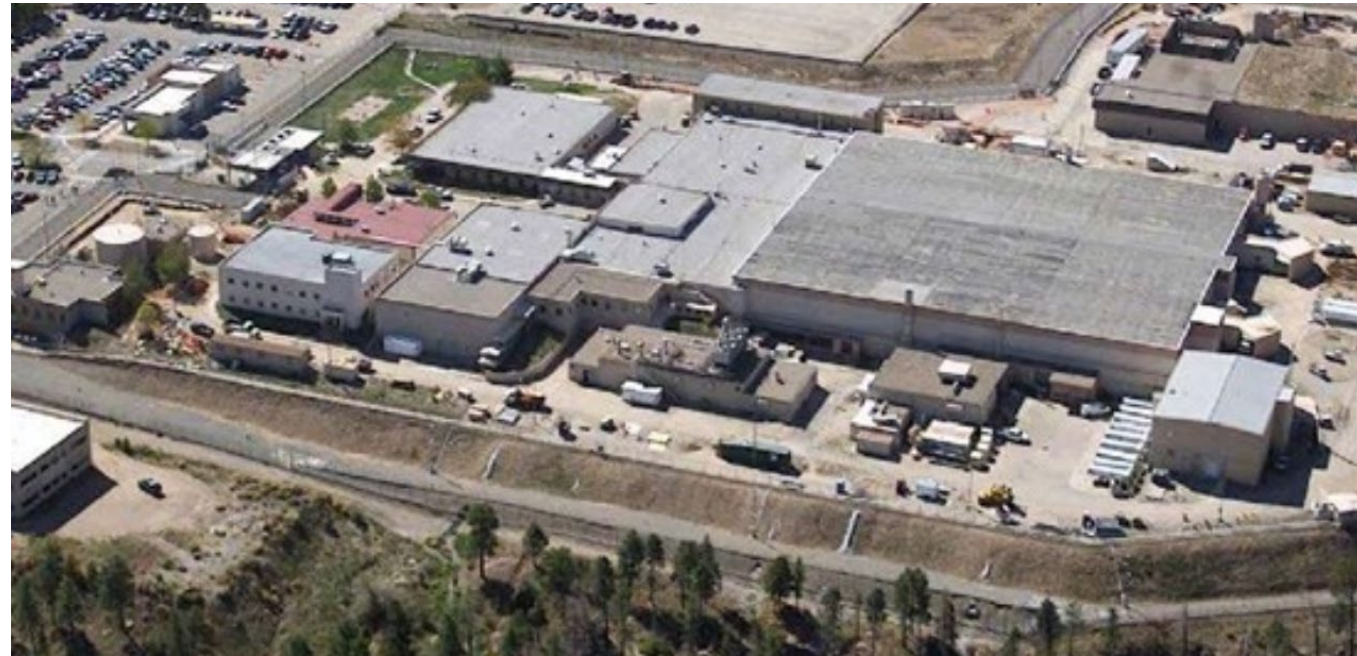
Aerial View of the Los Alamos Plutonium Facility
