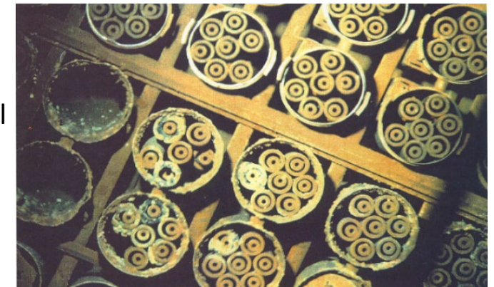
Spent fuel pool at Hanford K Reactor
