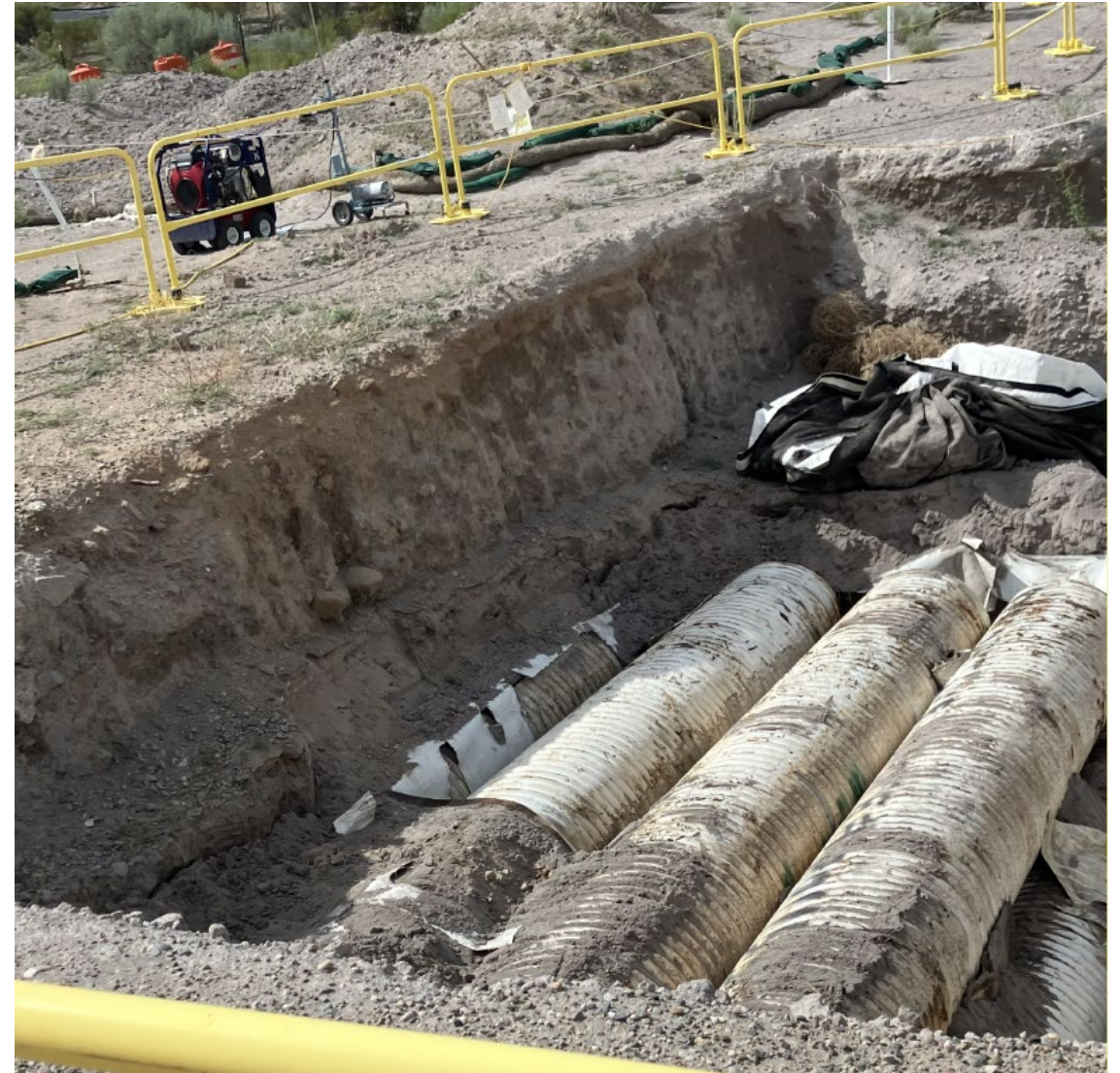
Excavation of Corrugated Metal Pipes
