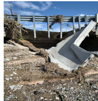
Highway 285 MM 88 bridge on Rio Felix Photo courtesv NMDOT
