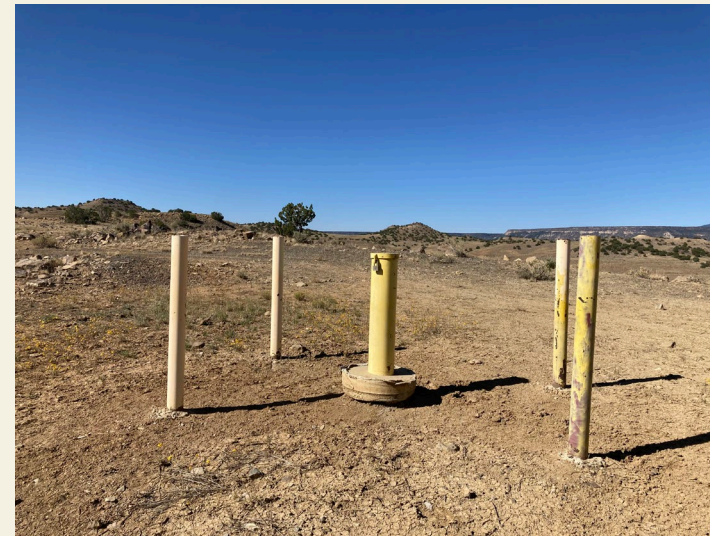
Monitoring well at J.J. No. 1 Mine
