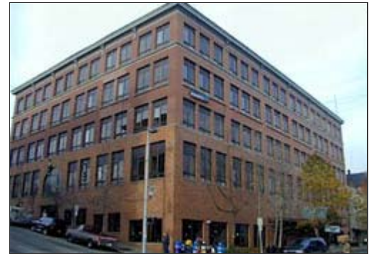
LCCA was among the many design and analysis tools used to transform this turn of the century building located in downtown Tacoma, WA into an energy efficient showcase building. (Courtesy of Washington State Department of General Administration)
