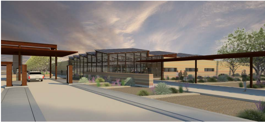
View of main building south side looking north
