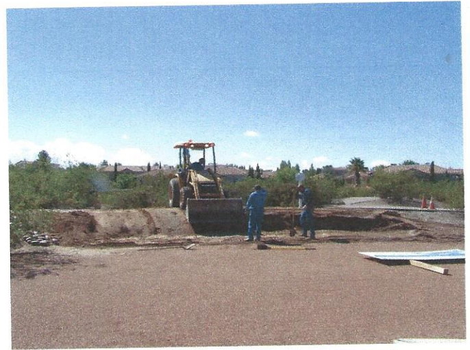
Clearing the ground August 2016
