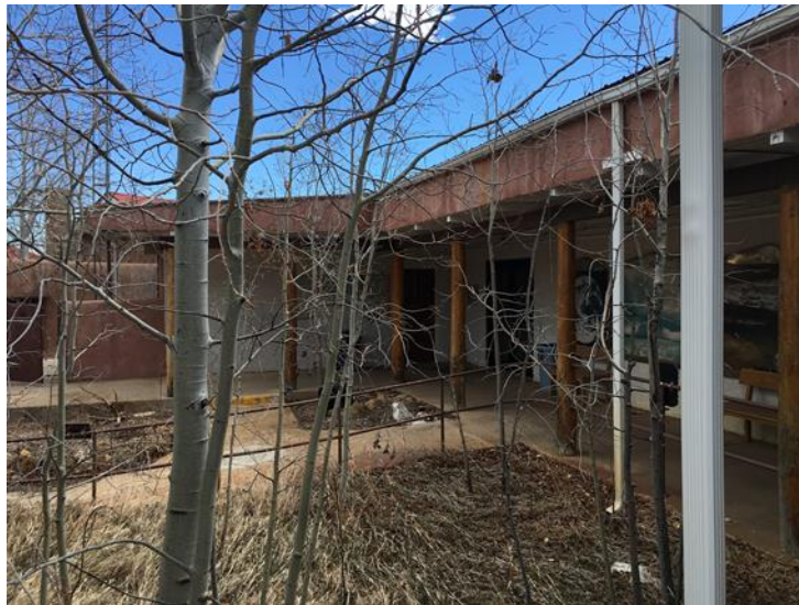
Exterior Portal facing the North
