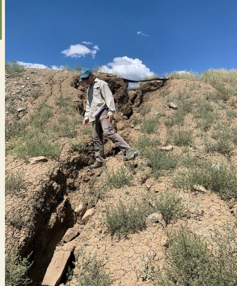
Erosion at J.J. No. 1 Mine
