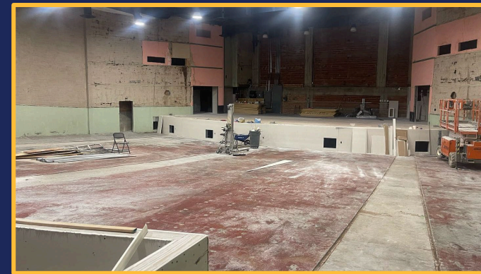
Cavern Theater Renovation: Digital Projection & Sound Total Project Cost: $5.2 million
