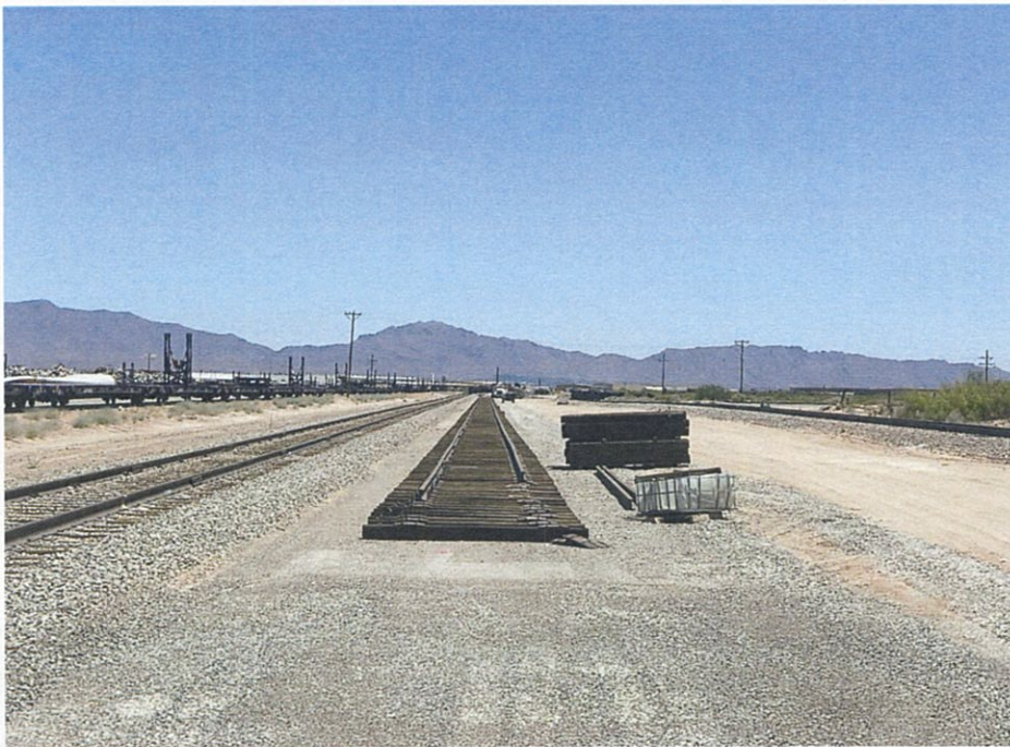
Track Construction in Progress
