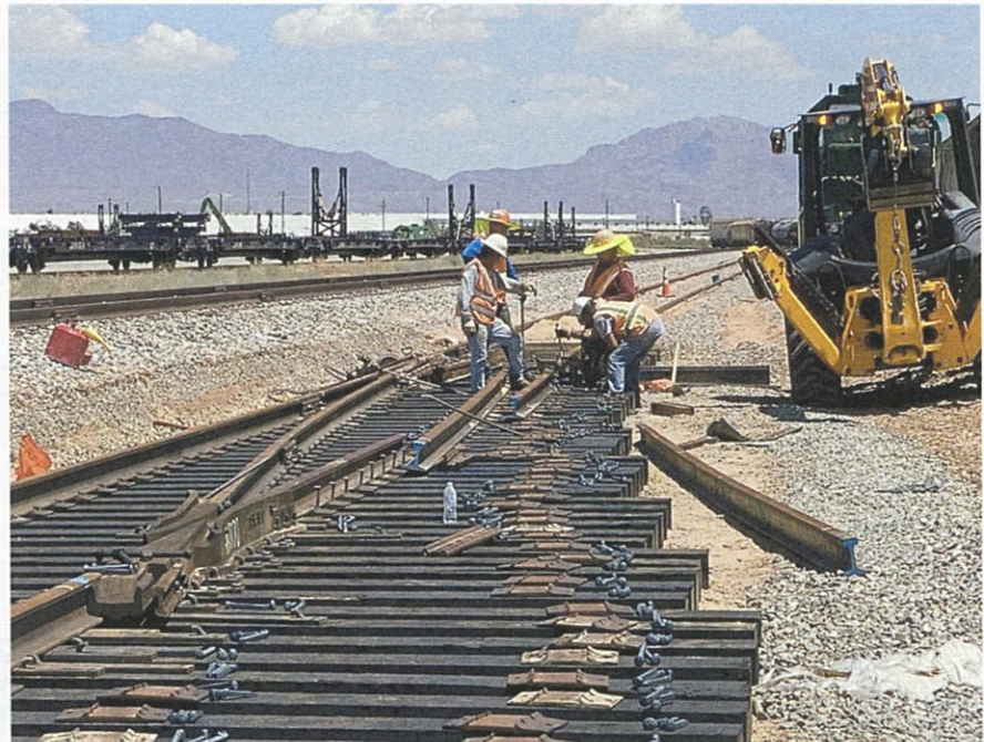
Rail Switch Installation in Progress
