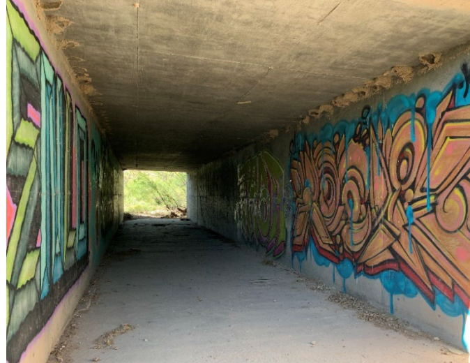
Figure 38: Box Culvert located on SLO property.
