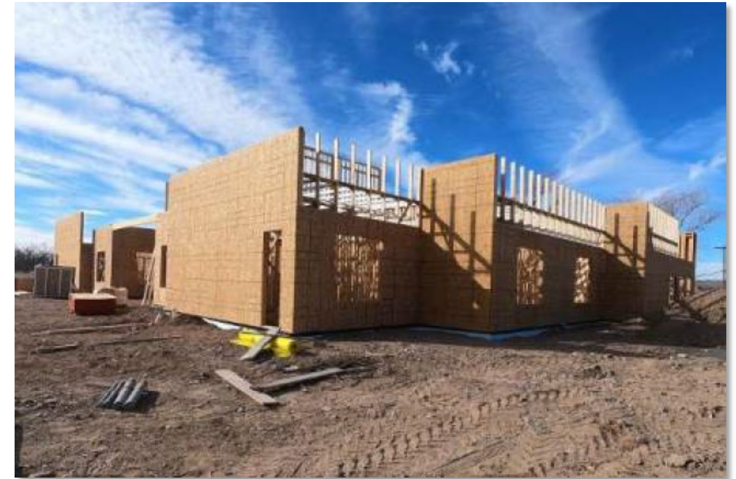
Small homes construction at New Mexico State Veterans Home, 11/30/22
