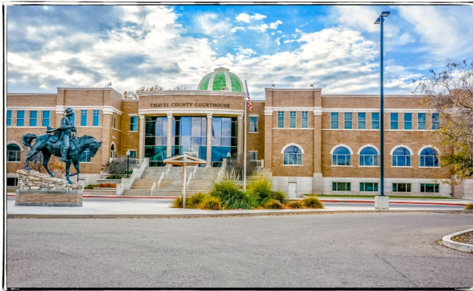
Chaves County Courthouse - newer construction
