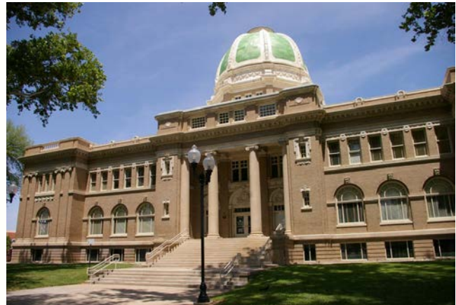
Chaves County Historical Courthouse - renovated
