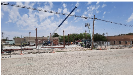
Lovington Magistrate Court construction site
