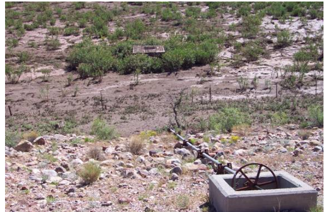
View of Outlet Gate Operator and Dry Reservoir
