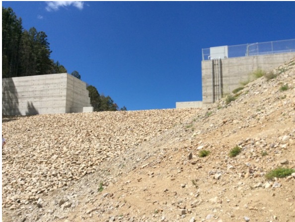
Site of New Dam
