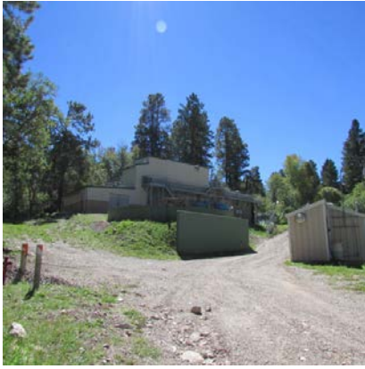
New Facility for Wastewater Treatment Plant
