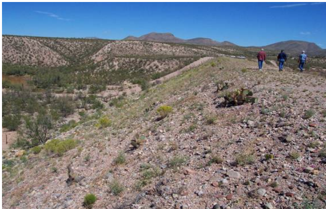
View of Upstream Dam Face with People Walking on the Dam Crest
