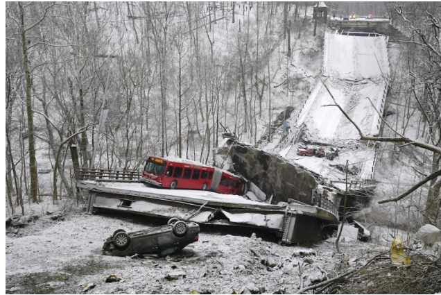
Pittsburgh bridge collapse Jan 2022
