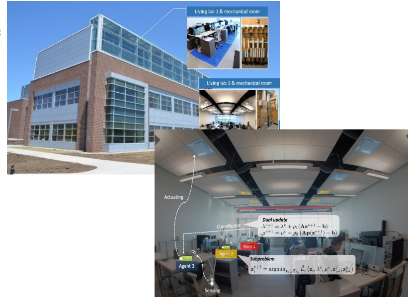
Purdue Living Laboratories with Retrofitted Air/Radiant Floor Systems
