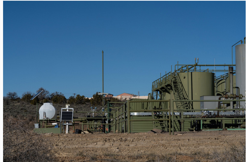
Oil and gas facility in Counselor, NM with Lybrook Elementary School in the background. Photo by Becca Grady.
