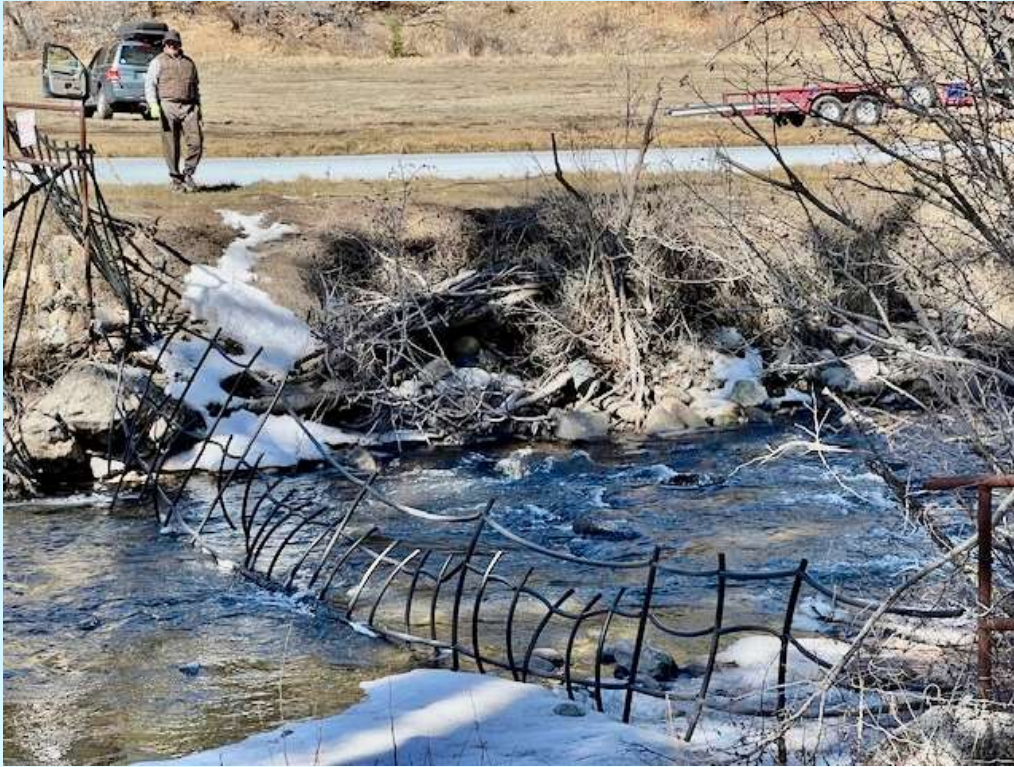
Fence on upper Pecos River prior to retrofit
