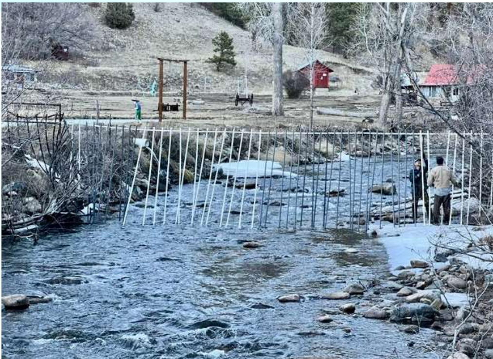
Retrofitted fence now paddler friendly
