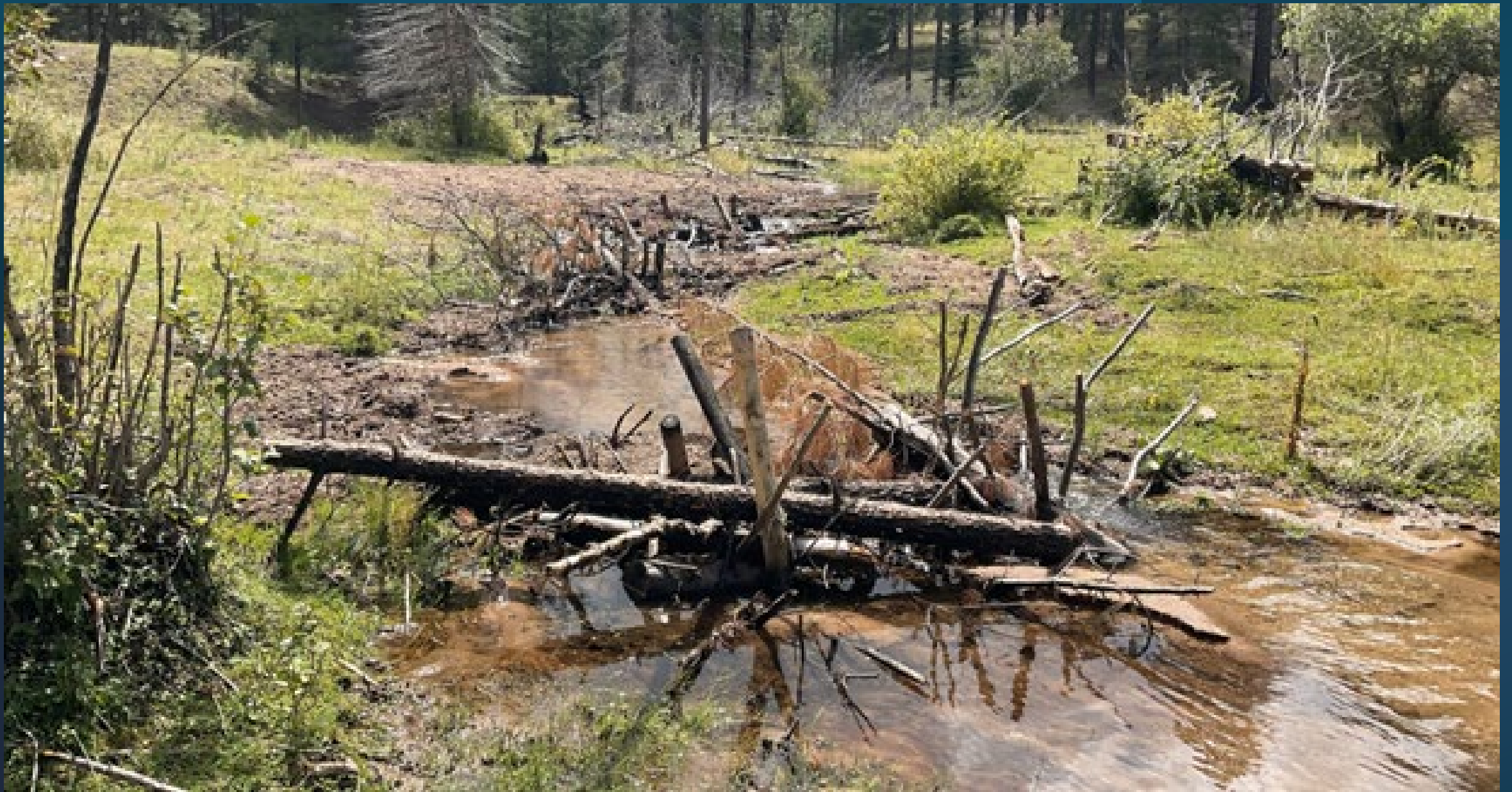
Post-Assisted Log Structure, Polvadera Creek
