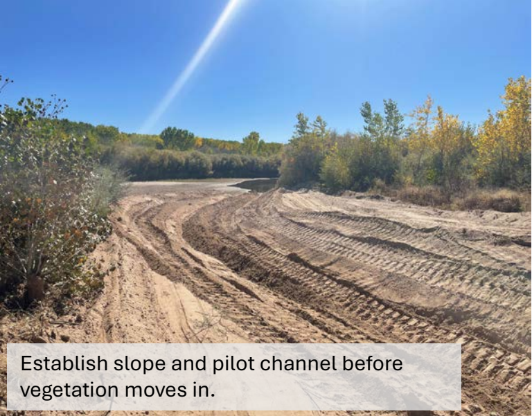
Send "pulse flow" through the pilot channel to mobilize and transport sediment out of the habitat feature with limited mechanical intervention.
