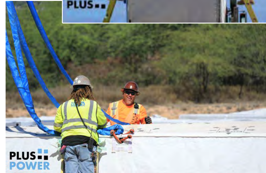
Kapolei Energy Storage – Oahu, Hawaii January 2023 Construction Photo
